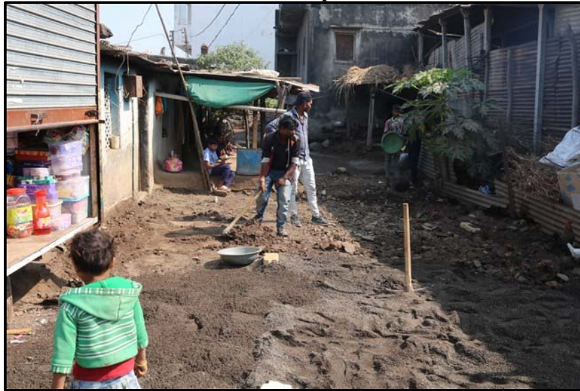
Image 4.5(A): Labourers (from Village) Constructing Pave-block Road, Mubarakpur
