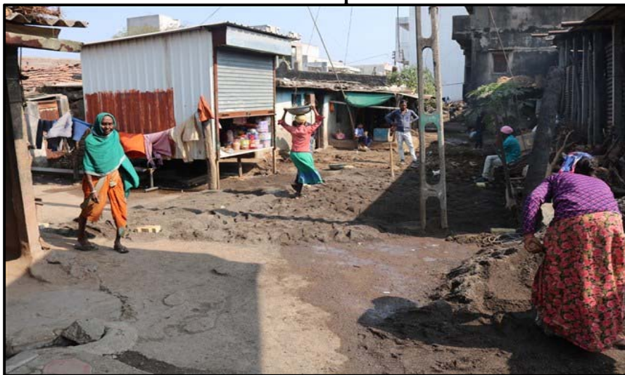
Image 4.5(B): Labourers (from Village) Constructing Pave-block Road, Mubarakpur
