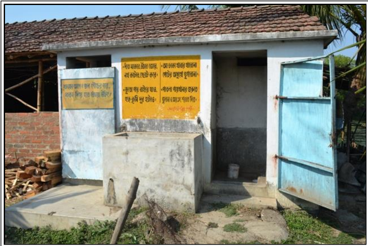
A toilet built under the Total Sanitation Campaign with wall-writing promoting behaviour change
