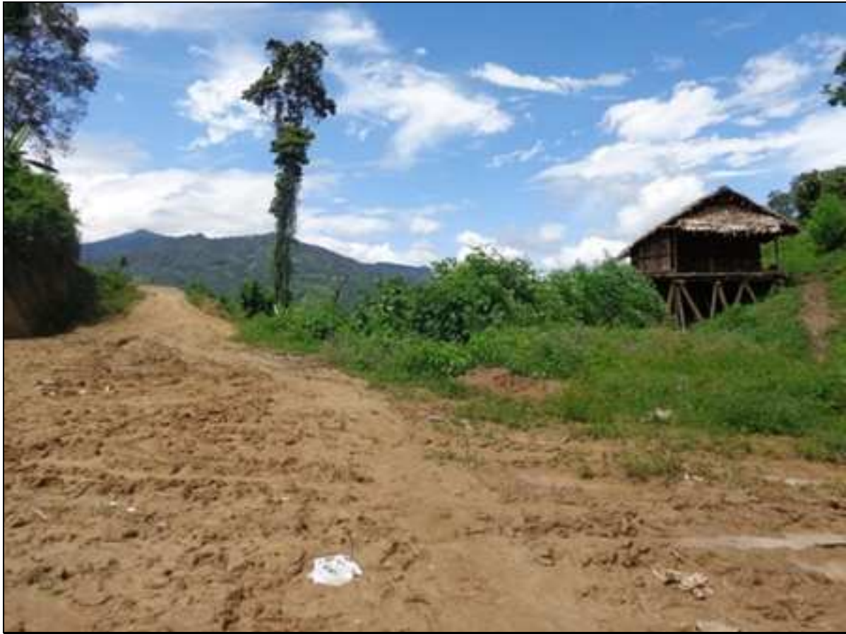
Photograph-- 9: Ambam-Silsango Road
