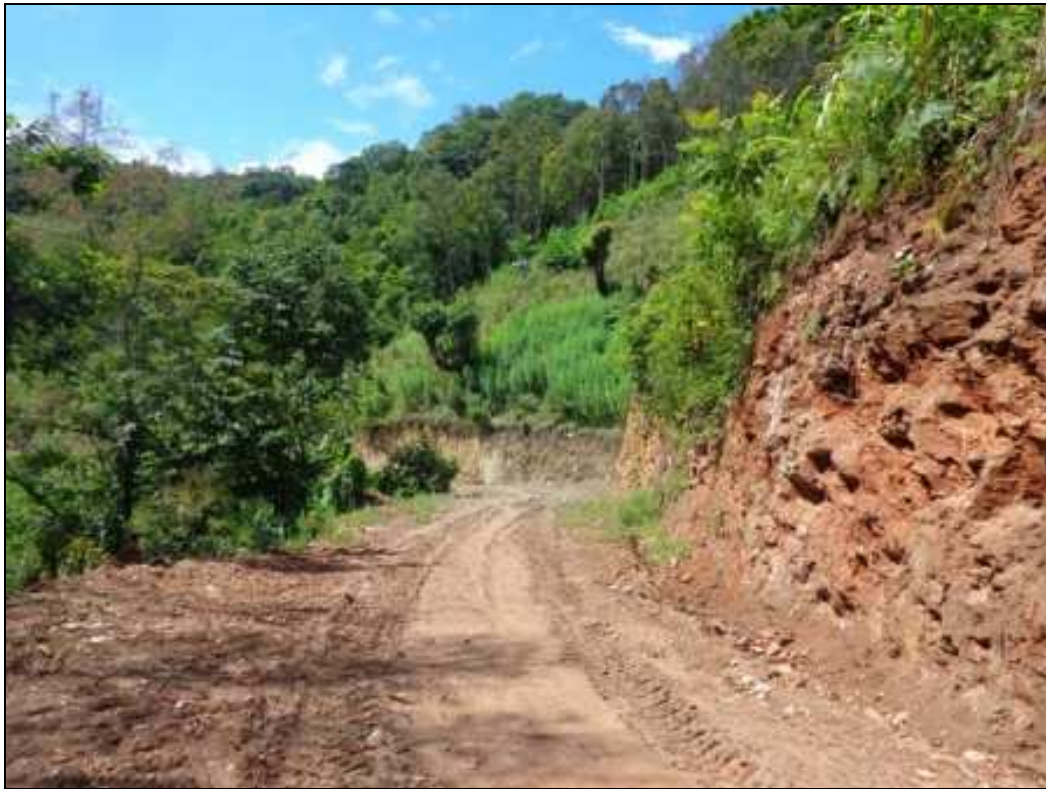
Photograph-- 6: Newly laid Ambam-Silsango Road
