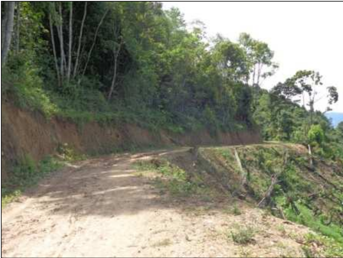
Photograph-- 7: Ambam-Silsango Road built by local Community
