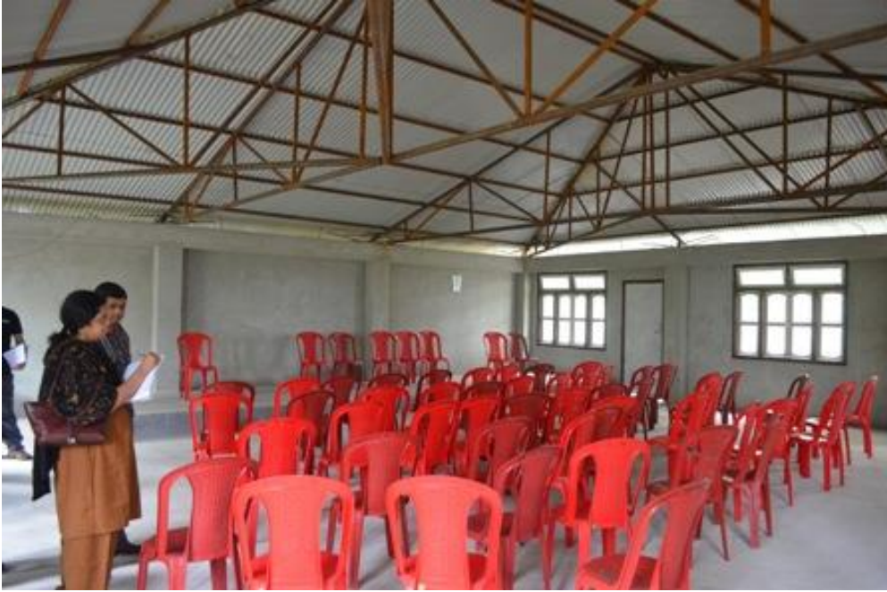
Photograph 6: Hall Constructed by GP for Gram Sabha
