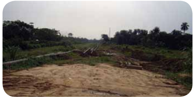
Gas pipelines run directly across agricultural fields, gardens and communal property.
