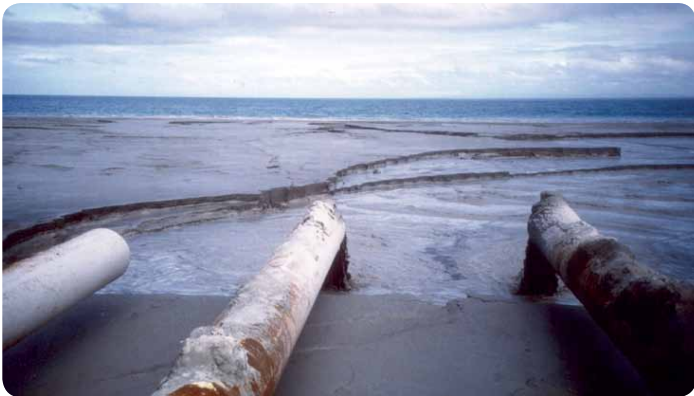
The Tapian pit pipes that transported tailings into Calancan Bay. PHOTO: Catherine Coumans.
