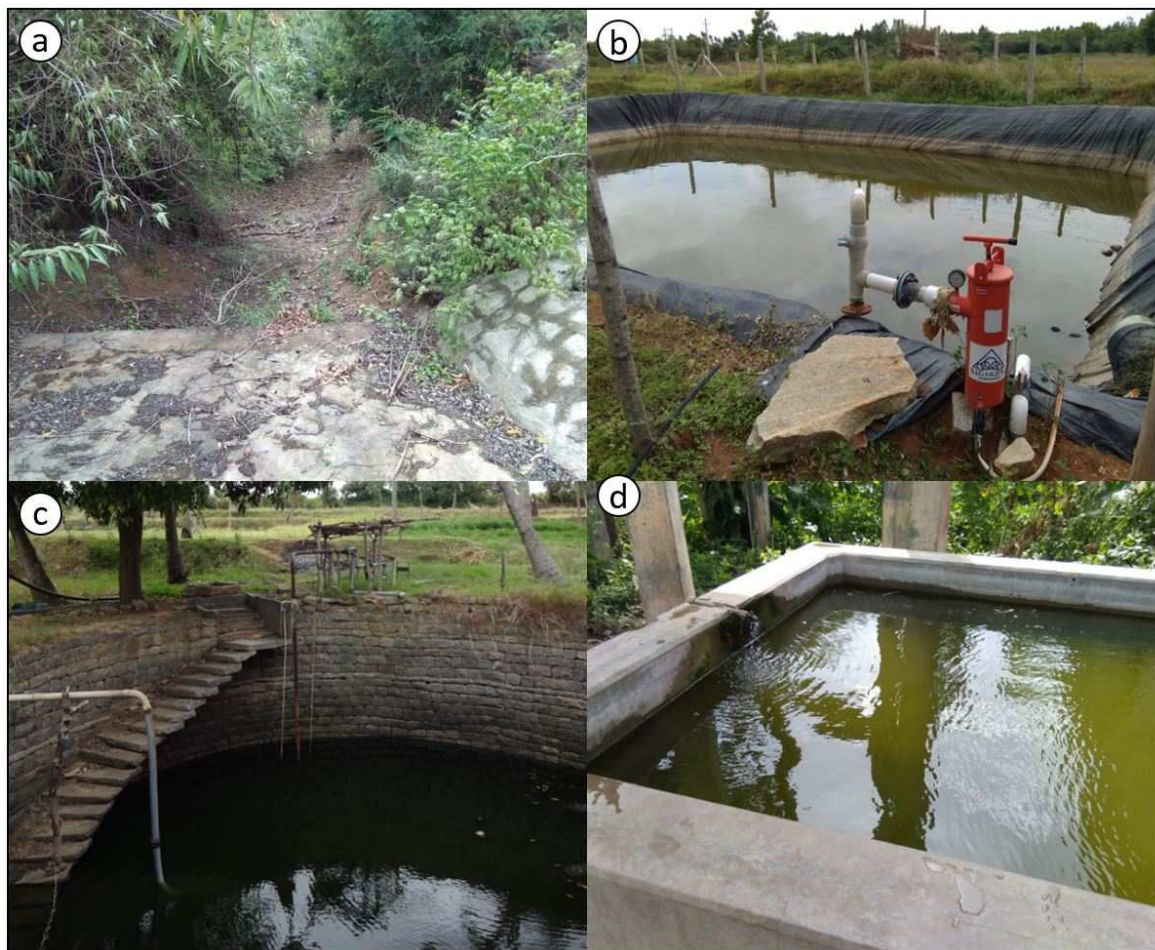
Figure 3. Water-holding structures created and encouraged as part of WSD projects: (a) check dam (without water); (b) farm pond (with tarpaulin lining); (c) open well; and (d) water trough for cattle (source: first author; images captured during transect walks in study villages).
