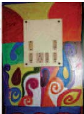
Beautifying a dirty switchboard
